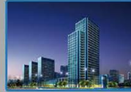
Networked Security: Building
